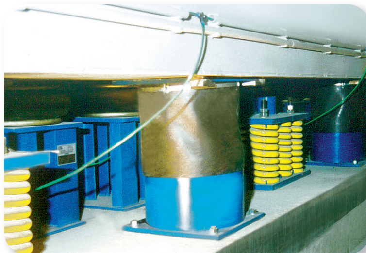
Steel springs under foundation
